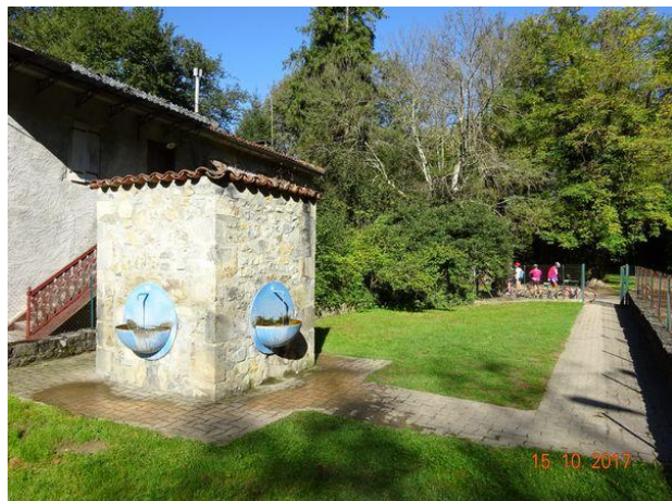
Sources de Ganties
